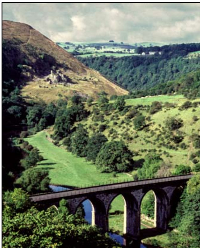
Monsal Dale and its distinctive old railway viaduct, as it was in the 1970s, with the limestone blocks and the head scar of the Hob's House landslide clearly visible on the hillside (photo: Tony Waltham).
